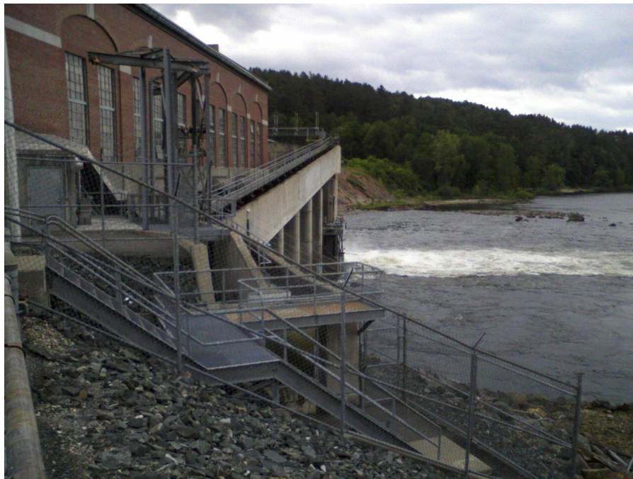
The Wilder Dam Powerhouse and fishway in Wilder, VT, 217 miles upstream of Long Island Sound. This is the most upstream dam on the Connecticut River that has a fishway for upstream passage of migratory fish. Two adult salmon tagged and released at Holyoke Dam have passed through this fishway this year. The spillway is on the other side of the powerhouse. The whitewater spill seen in the photo is provided for downstream passage of salmon smolts. The upper series of pools of the fishway is seen descending in front of the powerhouse. Below the superstructure is the countinghouse and window (can't be seen in this photo). The turn pool with a public viewing window is barely seen below the landing of the staircase. Then the fishway turns 180 degrees and descends down to the water level in front of the powerhouse, where there is an entrance gallery. The public viewing window is rarely opened to the public these days.
